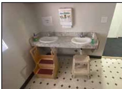
Sinks at wrong height for preschoolers
